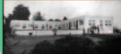
12 Second Loma Linda Hospital, August, 1924. The structure still stands as part of the west end of Nichol Hall.
